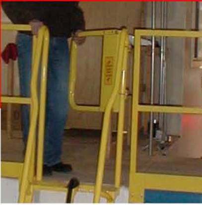
Powder Coat Safety Yellow Gate on an Alternating Tread Industrial Stair.
